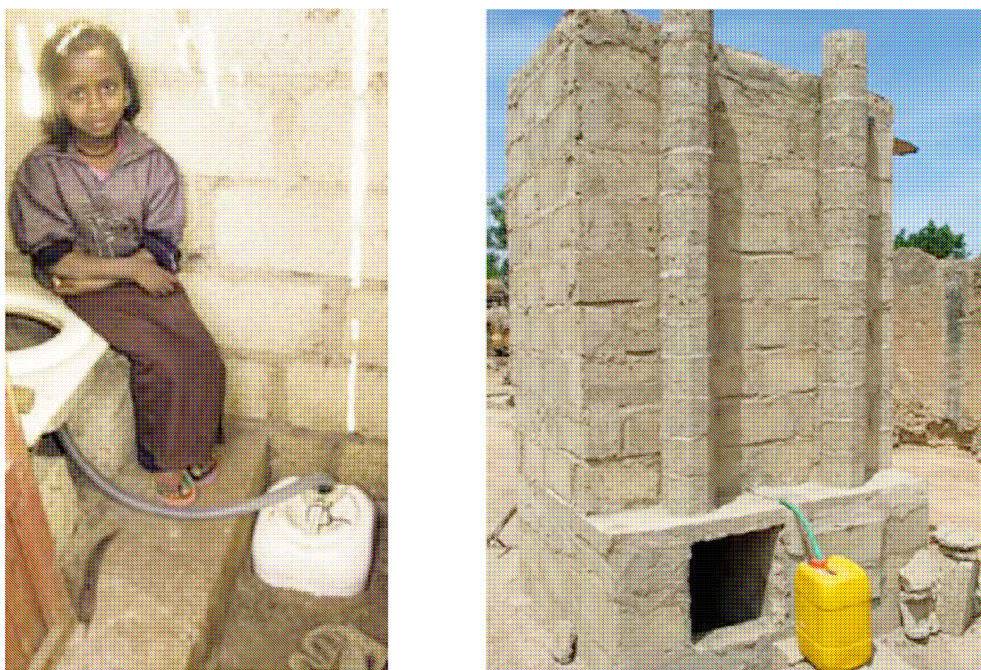
Figure 32: Urine diversion toilet in Ethiopia (left) 9 and in Burkina Faso (right) [41]
