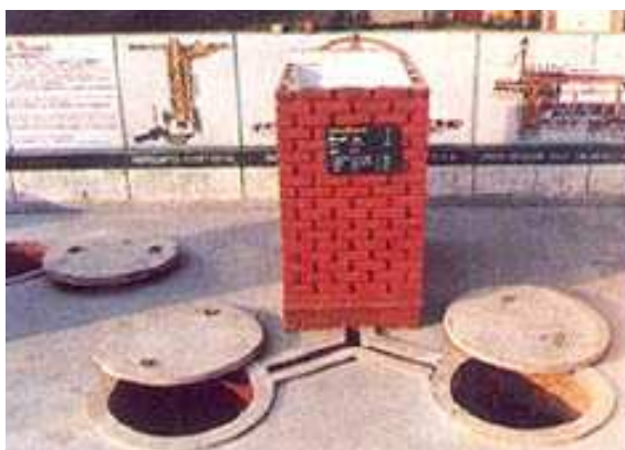
Figure 46: Two-pit pour-flush Sulabh toilet [ www.sulabhinternational.org ]
